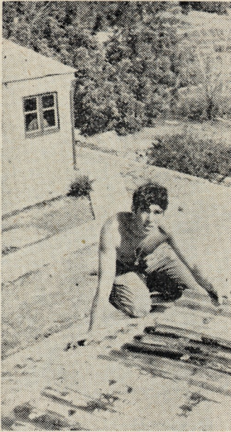
● Corporal Fred Fielding carries out repairs on the Medical Centre.
