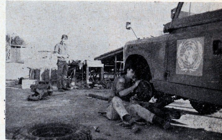
● Private John Murphy adjusts brakes while in the background Private Paddy Bradshaw works away.
